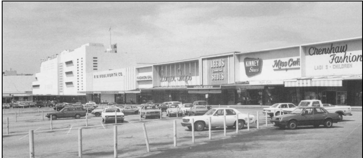
Broadway-Crenshaw, Los Angeles, CA, shortly before demolition. (Richard Longstreth).
